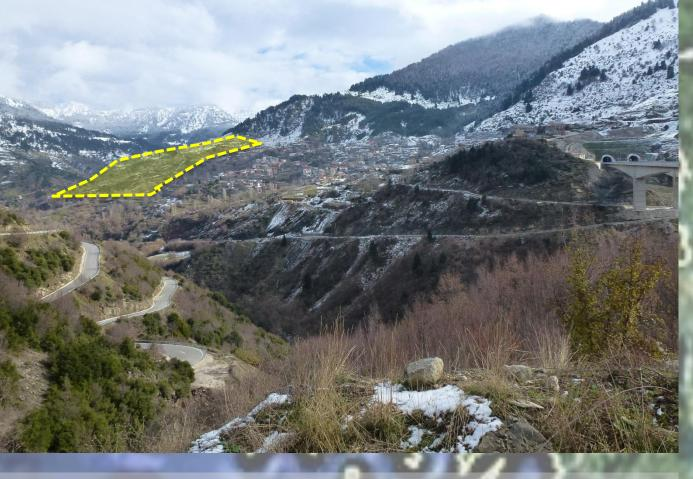
The final location of the Aniliou tunnel shown above had to be relocated due to a landslide in the original alignment. The approximate limits of the slide mass are outlined in yellow The tunnel was moved behind the instability into the more competent rock mass behind.
