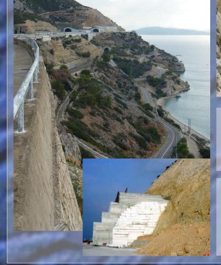
Twin highway tunnels were conventionally excavated parallel to the 15 – 20 km long active Kakia Scala fault system, in karstic limestone. The tunnels have been designed to allow for 0.3 to 0.5m of vertical movement along the fault plane.
