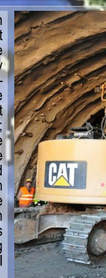
Due to substantial weathering of molasse at surface, heavy support is required in the portal area. The photo above shows installed support including: steel sets with elephant feet at 1m spacing, 25cm of shotcrete, 6m grouted rock bolts, and 6m long, grout-filled forepoles. As the effects of surface weathering reduce with depth, and rock quality improves, support requirements will be decreased.
