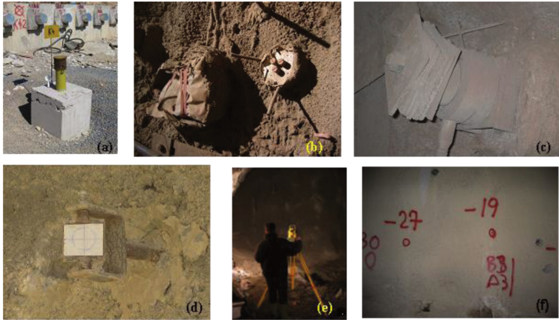
Fig. 12. Optical survey markers and their locations within the tunnel excavation. Note that A-Phase and B-Phase are analogous to top heading and bench excavation phases, respectively.
