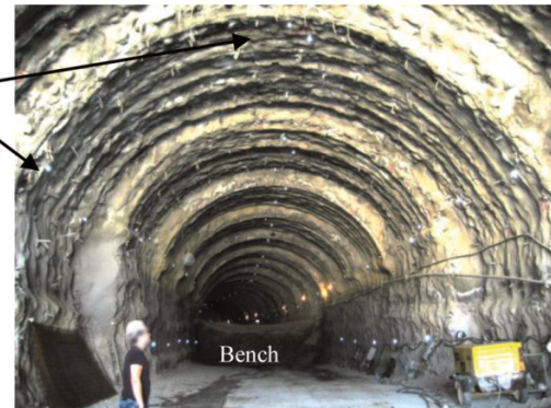
Fig. 12. Optical survey markers and their locations within the tunnel excavation. Note that A-Phase and B-Phase are analogous to top heading and bench excavation phases, respectively.
