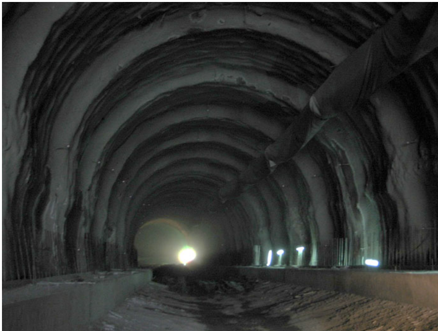
Fig. 20 “Saw-tooth” profile of the umbrella arch installed in the Driskos tunnel
