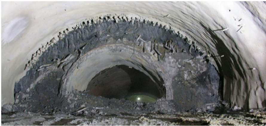
Fig. 17 Over excavation of the pilot tunnel in the south bound tunnel, December 2012
