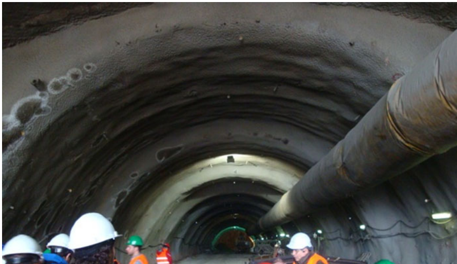
Fig. 15 Platanos tunnel section during a site visit by the authors in December 2010
