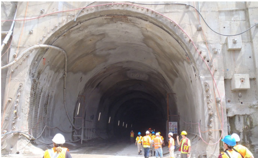
Fig. 18 Tunnel San Fedele (Roveredo bypass project) south portal during a site visit by the authors in 2011
