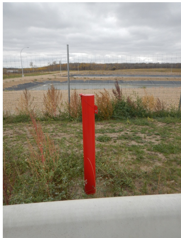
Figure 35: New Effluent Lagoon Monitoring Well – Point 5
