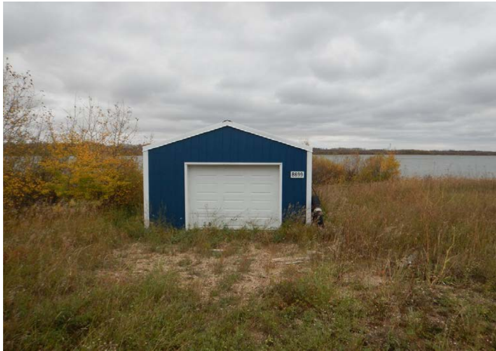
Figure 15: Pump Station – Houses Manhole – Fish Kill Location – Point 4
