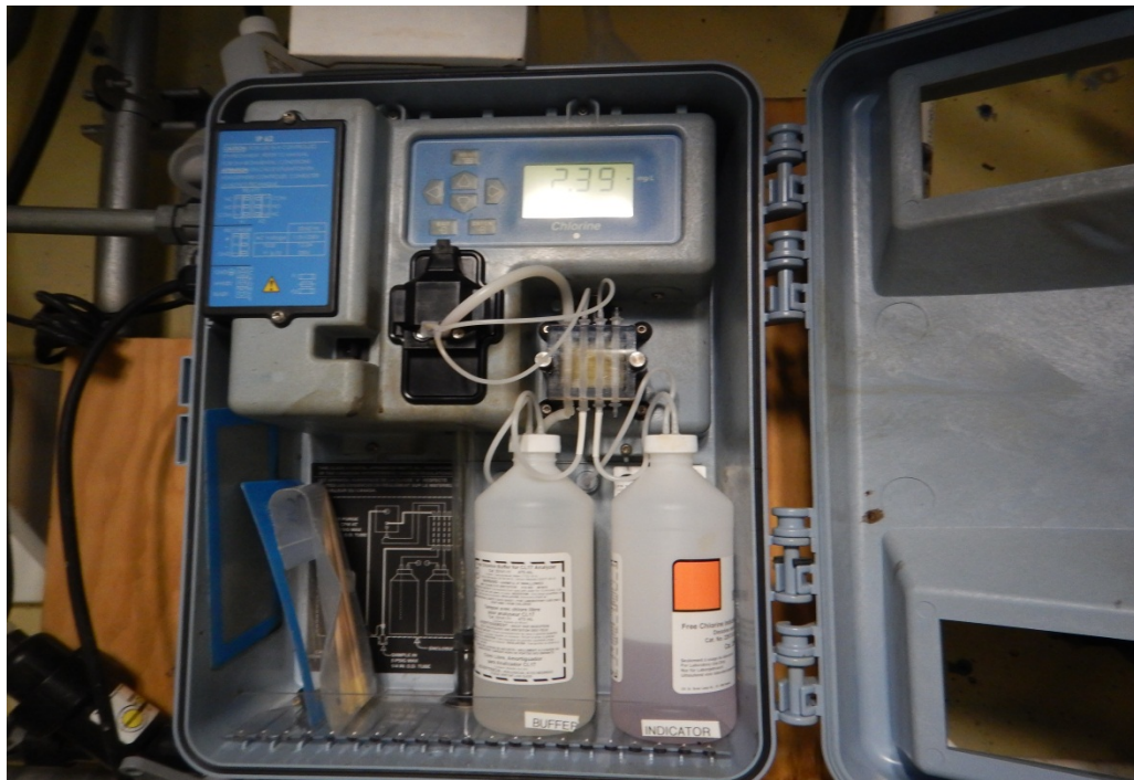
Figure 27: Chlorine Monitor – WTP
