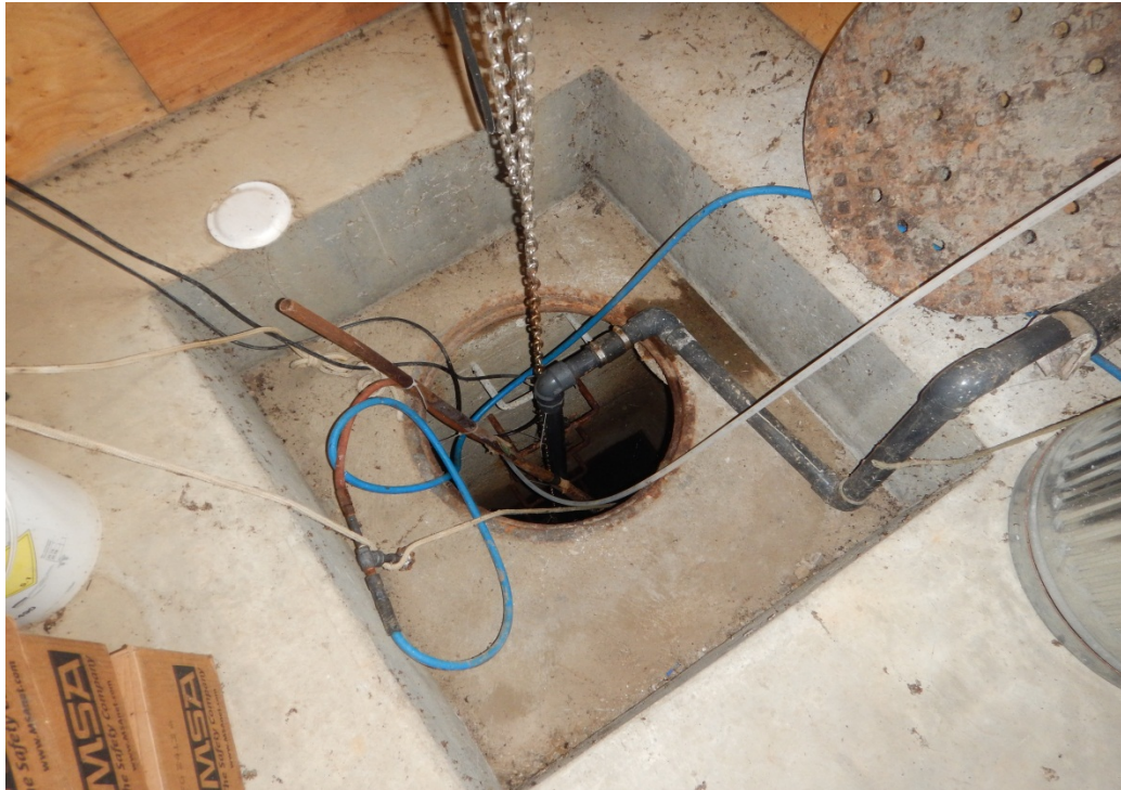
Figure 34: Manhole Pump Station – Betty Lake – Point 4
