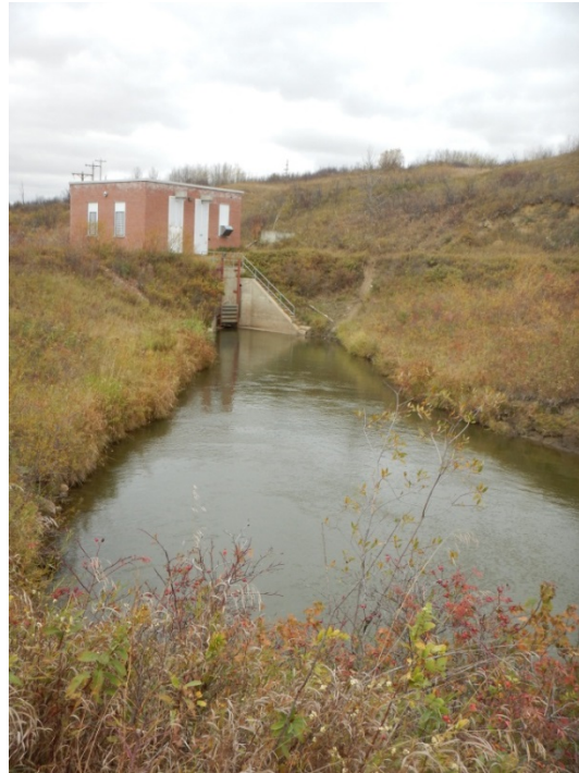
Figure 54: Battle River Intake – Pump House and Intake Channel - Point 7
