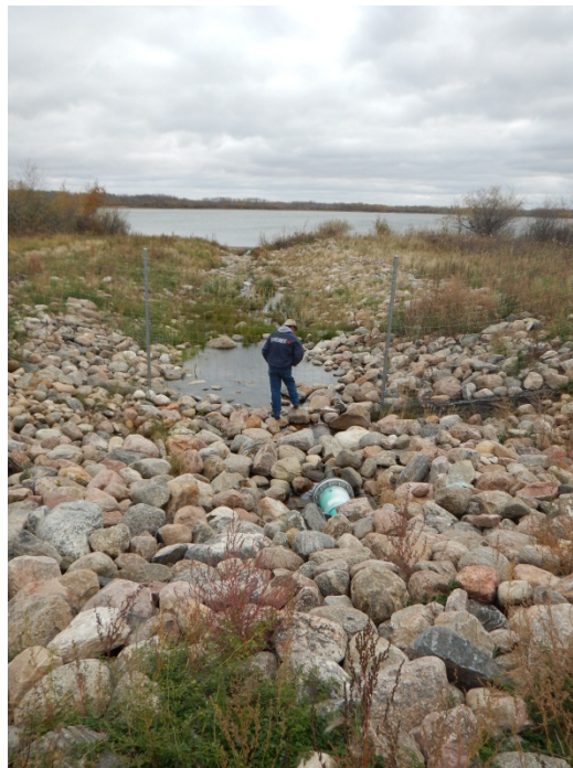
Figure 49: New South Effluent Lagoon - Effluent Pipe to Betty Lake – Point 6
