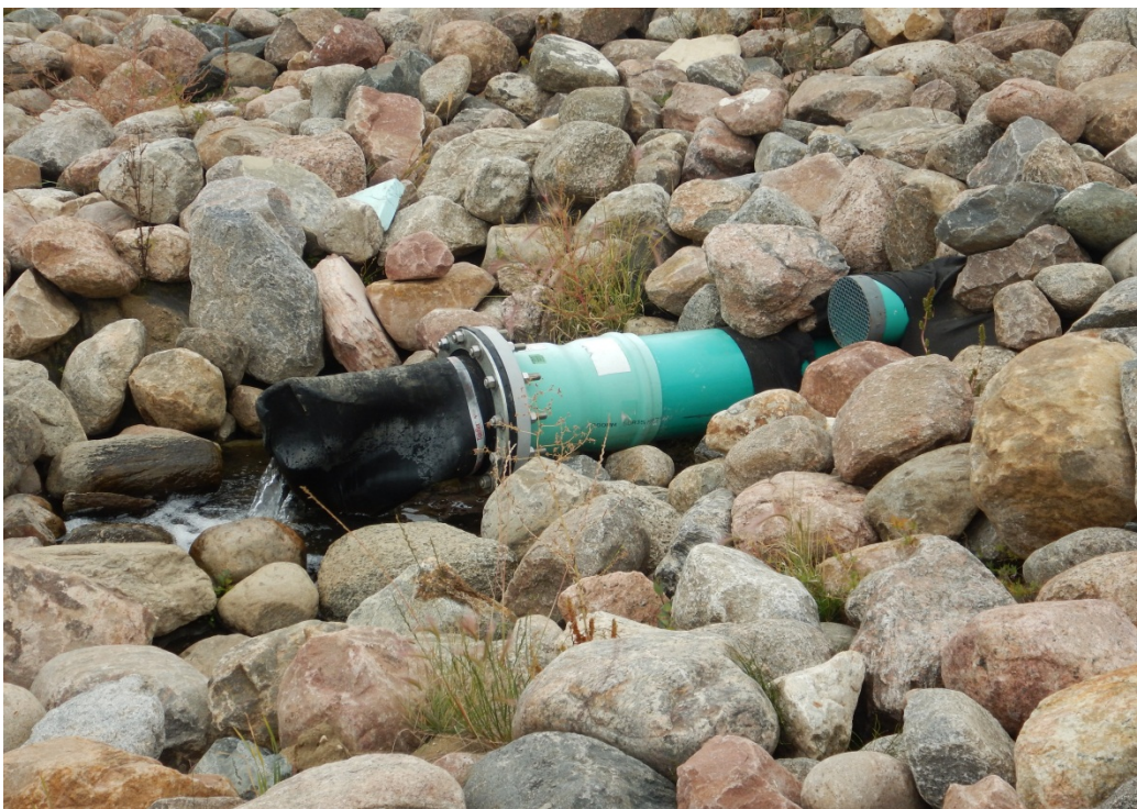
Figure 39: New South Effluent Lagoons – Effluent Pipe to Betty Lake with Barrier – Point 6
