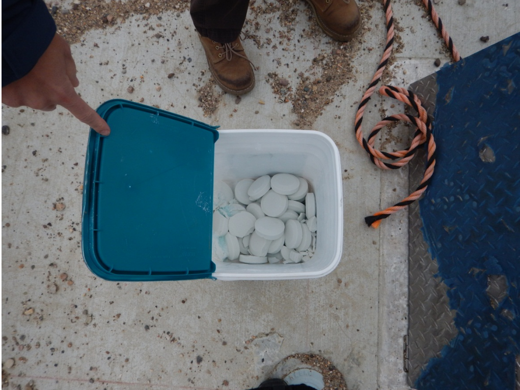
Figure 40: New Effluent Lagoon – Dechlorination Tablets – Point 6
