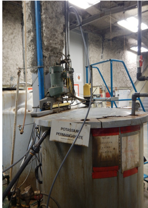
Figure 20: Potassium Permanganate Container - WTP
