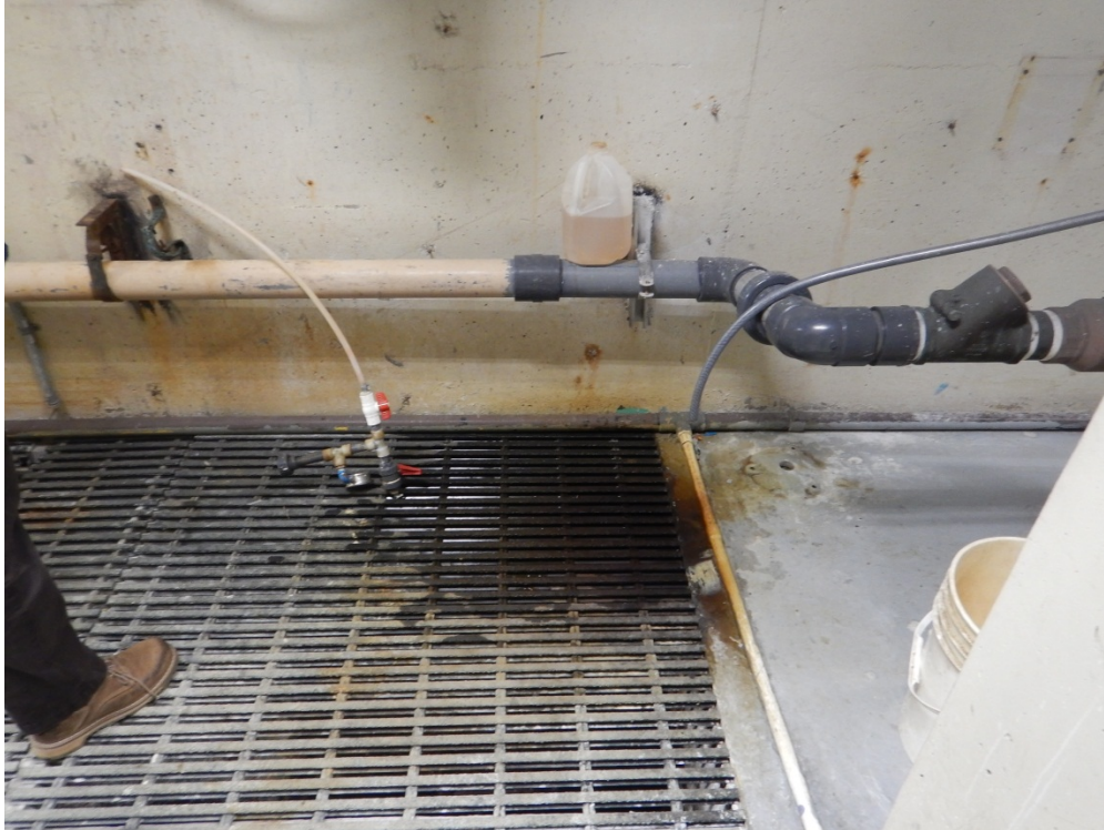
Figure 24: Leakage – WTP
