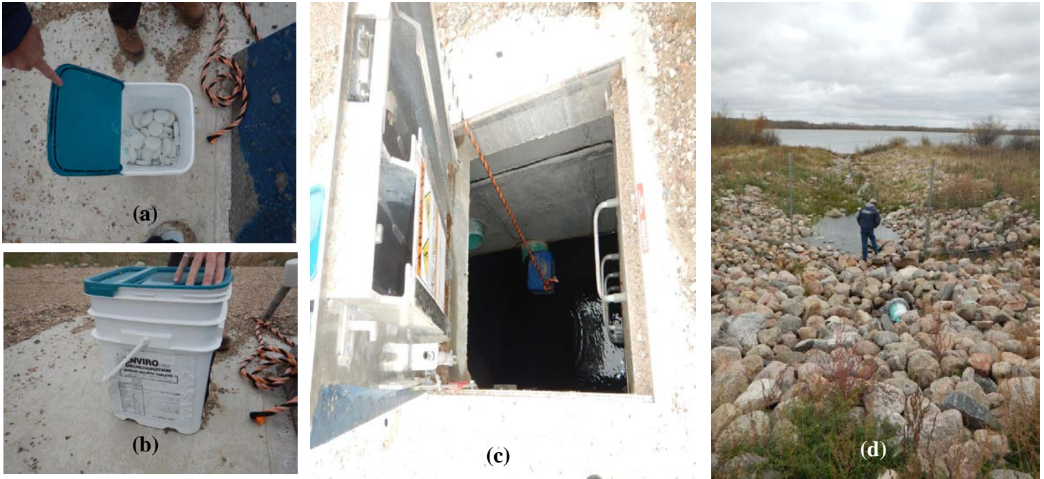
Figure 10. Dechlorination Process at South Lagoon (photos taken in October 2014 by RMC Green Team). (a) Dechlorination ‘pucks’ or tablets, (b) container of Sodium Sulphite Tablets, (c) Manhole at the effluent culvert from the South Lagoons depicting the perforated container that is filled with dechlorination tablets and placed at the culvert opening and, (d) exiting side of the effluent culvert that discharges to Betty Lake towards the East (in the background)
