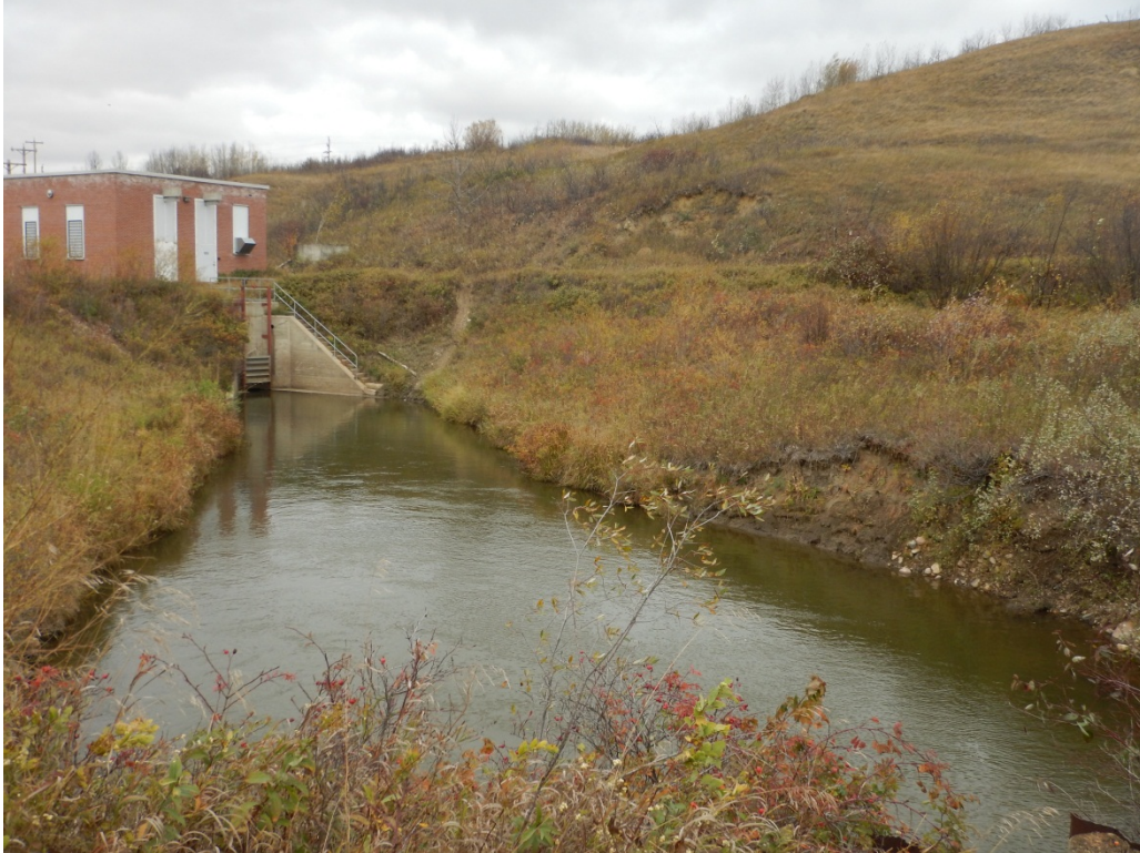
Figure 56: Battle River Intake - Pump House and Intake Channel - Point 7
