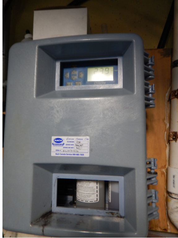
Figure 26: Chlorine Monitor – WTP
