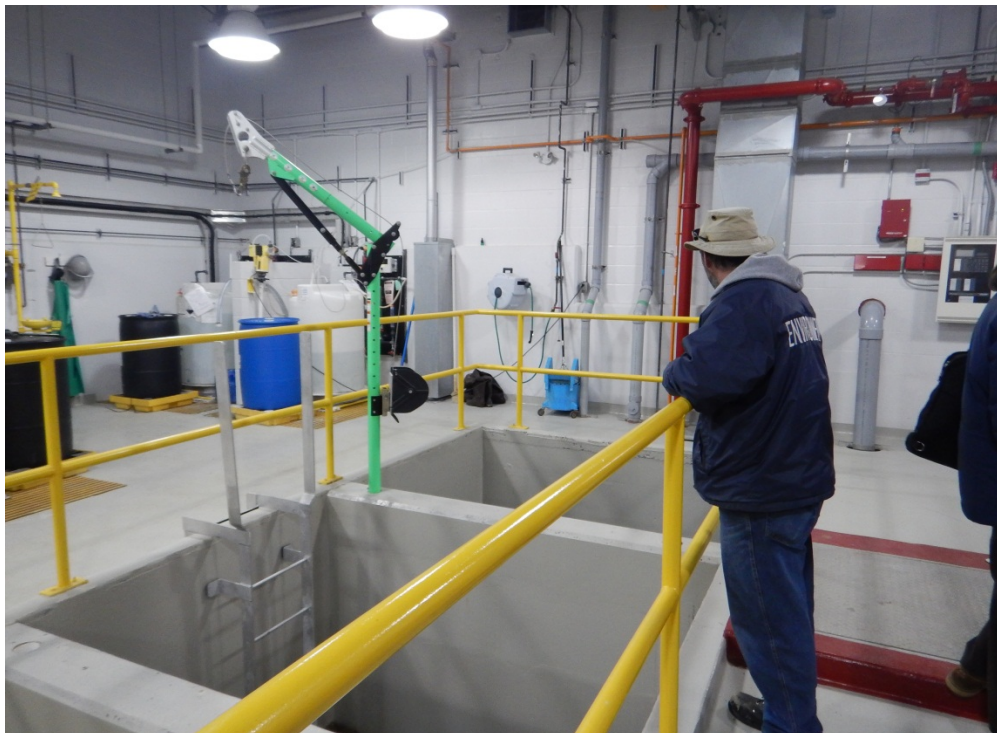
Figure 31: New Filters – WTP
