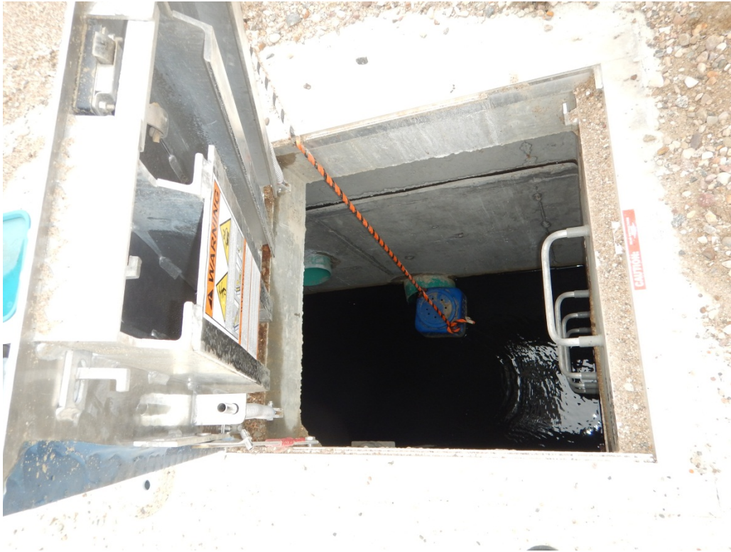
Figure 42: New South Effluent Lagoon - Effluent Pipe Manhole to Betty Lake – Point 6
