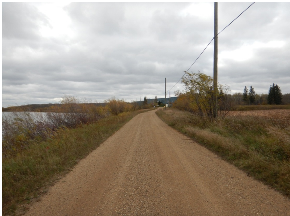
Figure 14: Causeway Facing Plant (NE) - between Pts 2 and 3
