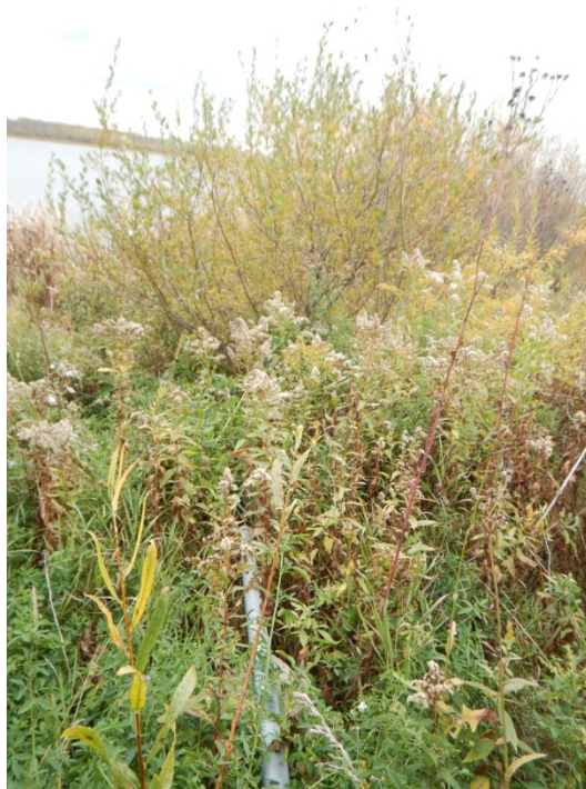
Figure 17: Pump Station Pipe – Effluent – Fish Kill Location – Point 4
