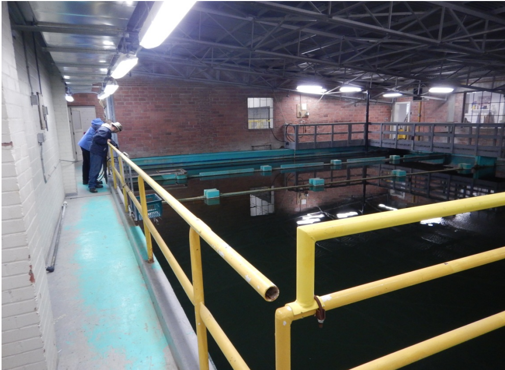
Figure 30: Settlement Tanks – WTP
