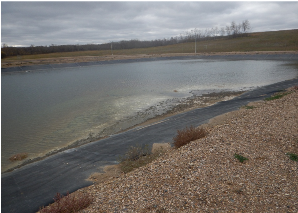
Figure 37: New South Effluent Lagoons – Geomembrane Liners – Point 5
