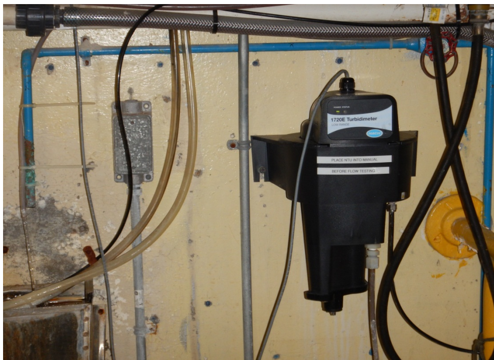
Figure25: Turbidimeter – WTP
