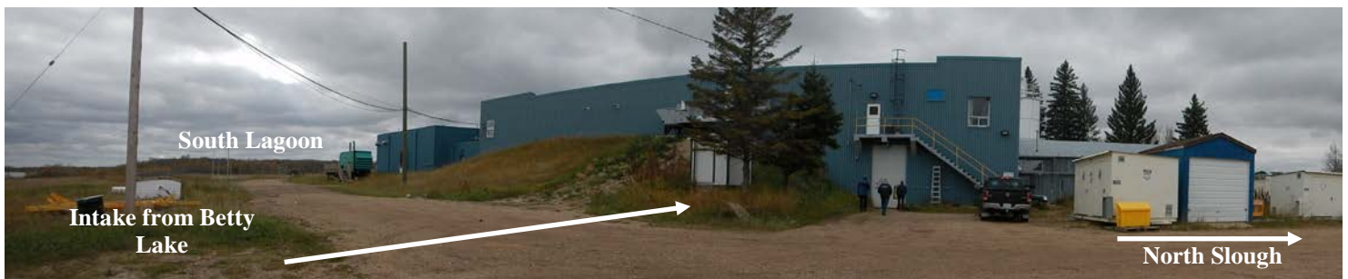
Figure 9. Photo of WTP facing north. More Photos and site map in Annex A .
