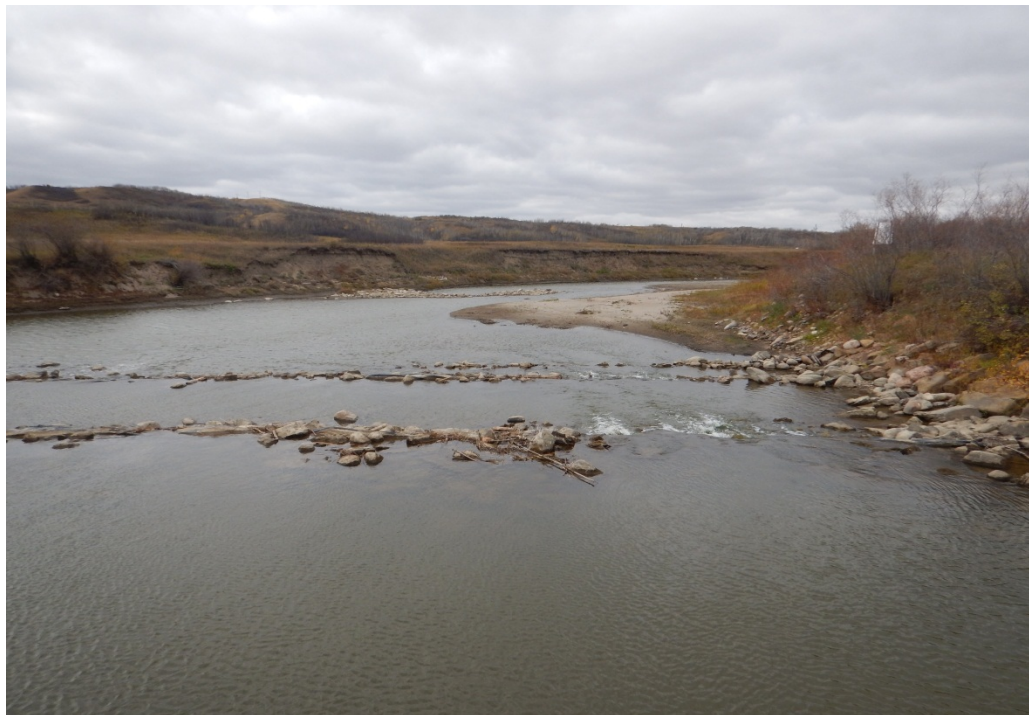
Figure 53: Battle River Intake – Facing North - Point 7
