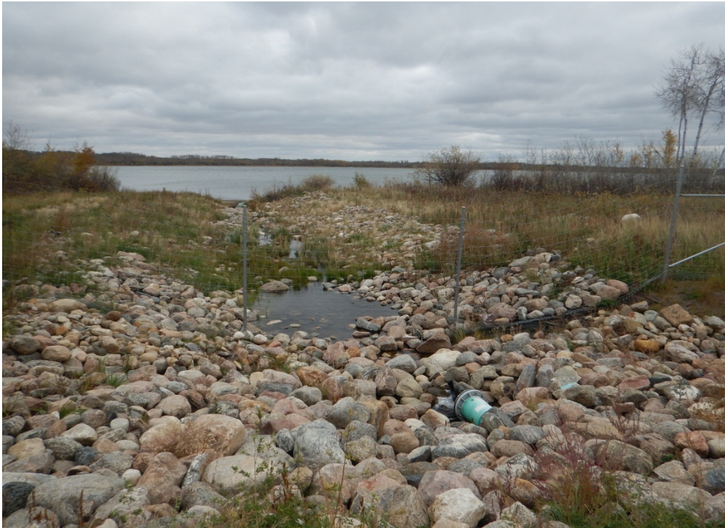
Figure 38: New South Effluent Lagoons – Effluent Pipe to Betty Lake – Facing East - Point 6
