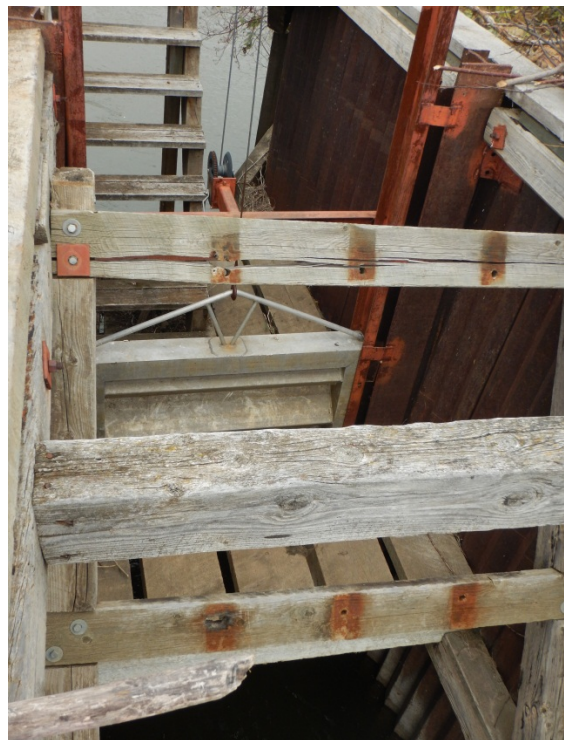
Figure 55: Battle River Intake Channel - Point 7
