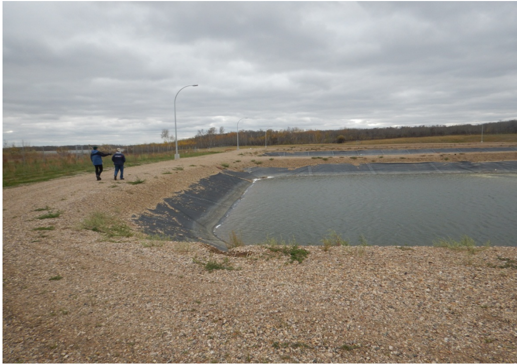
Figure 36: New South (Effluent) Lagoons – Facing South West - Point 5
