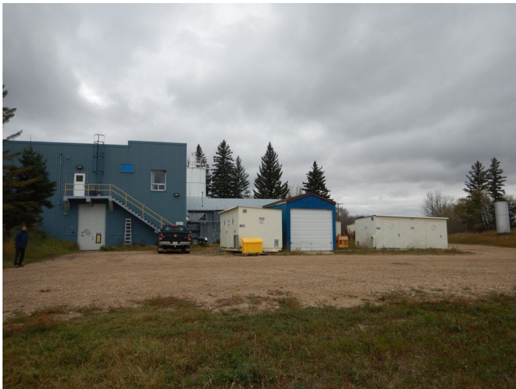
Figure 18: WTP – Storage and New Extension – Point 4 facing North
