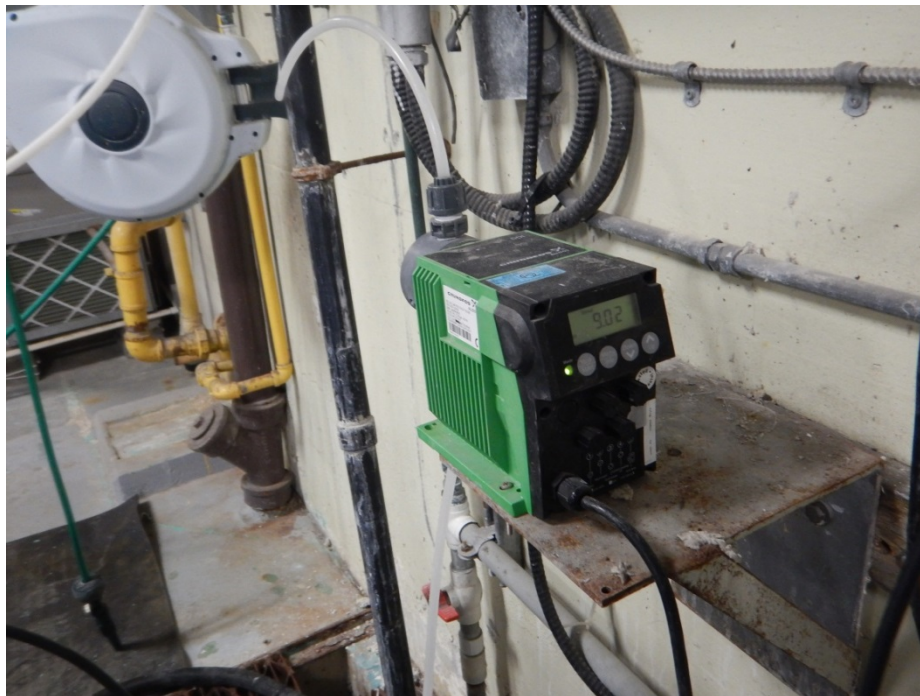
Figure 21: Potassium Pump - WTP
